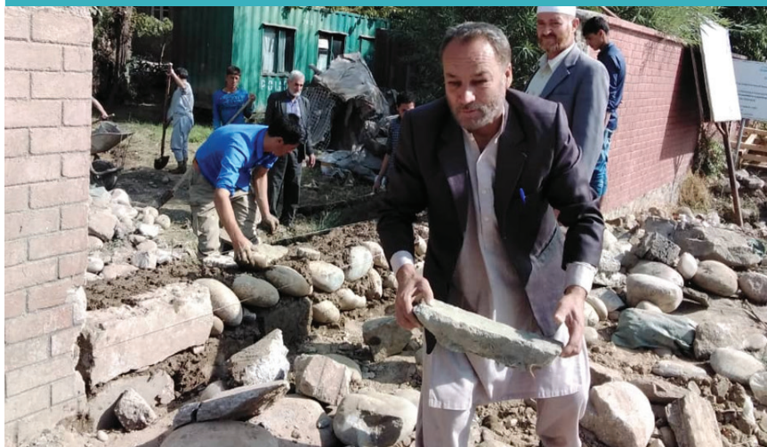
Figure 3. Mirmasjidi High School (October 2020), Kapisa province: repair work on the school perimeter wall.
